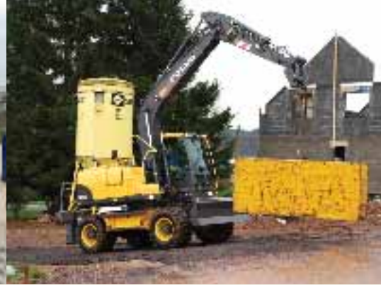
• Reach and power for lifting and placing.
